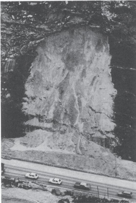
Figure 5. Typical Hong Kong soil cut slope failure caused by heavy rainfall
